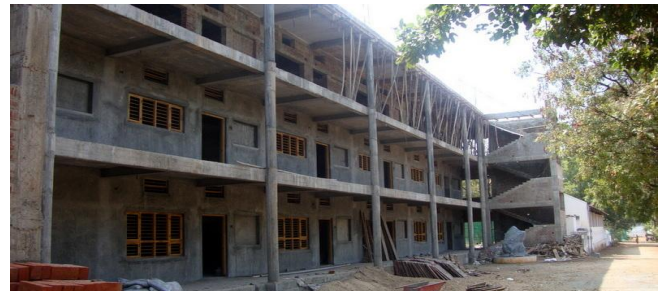
A view of the new building under construction
